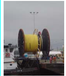
J P Kenny provides installation Engineering and supervision services for deepwater systems
