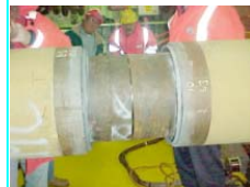
"Welding of Pipe-in-pipe system"
